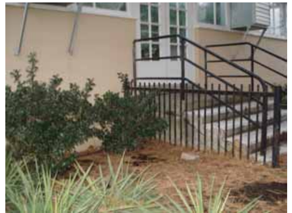
Figure 6- Play Area – prickly bushes/spike/poky plants; thick mulch could prevent seeing clearly items that should not be in children's play areas
