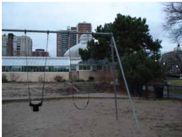
Figure 7 Playground Area – paved path raised along edge of sand area; on other side of path is a concrete slope surrounding wading pool's open south side; curb is a tripping problem; path does not provide surface for strollers, wheel chairs, tricycles
