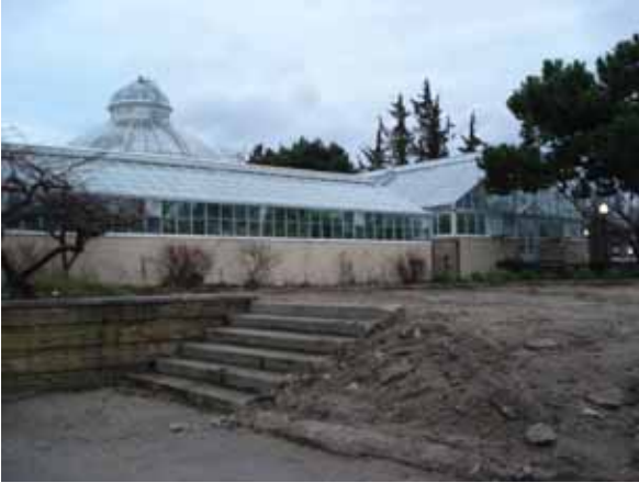
Figure 5-Concrete Steps – dangerous for all patrons of the park
